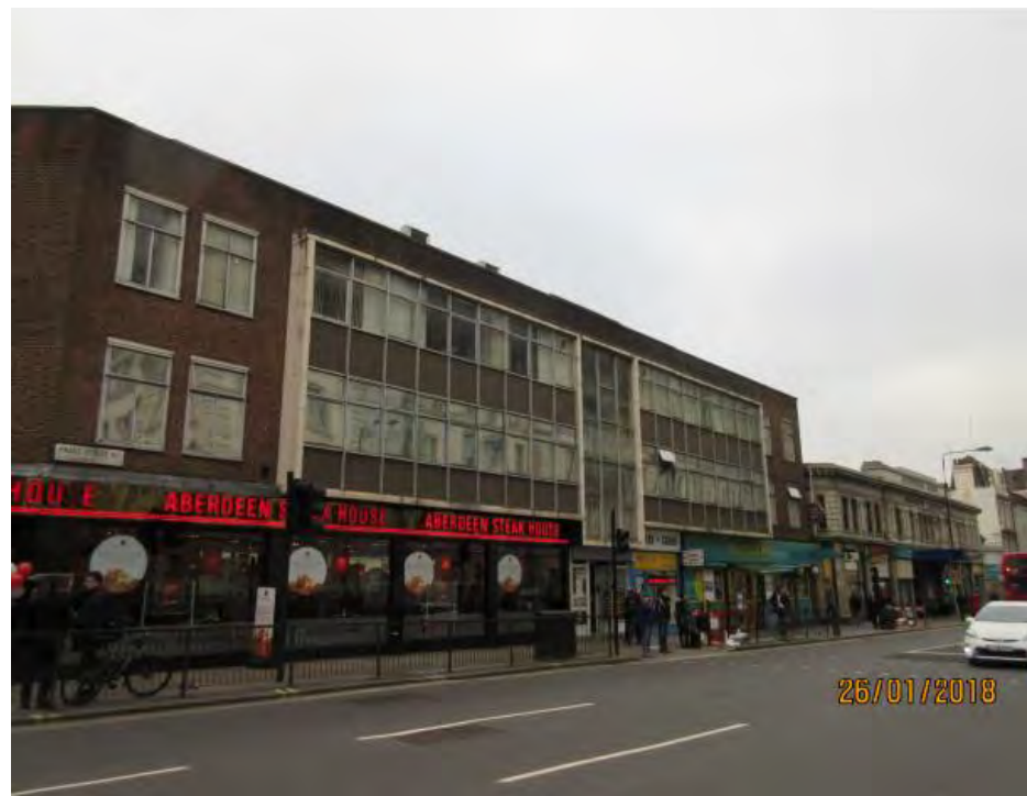
Views of existing building from Praed Street.
